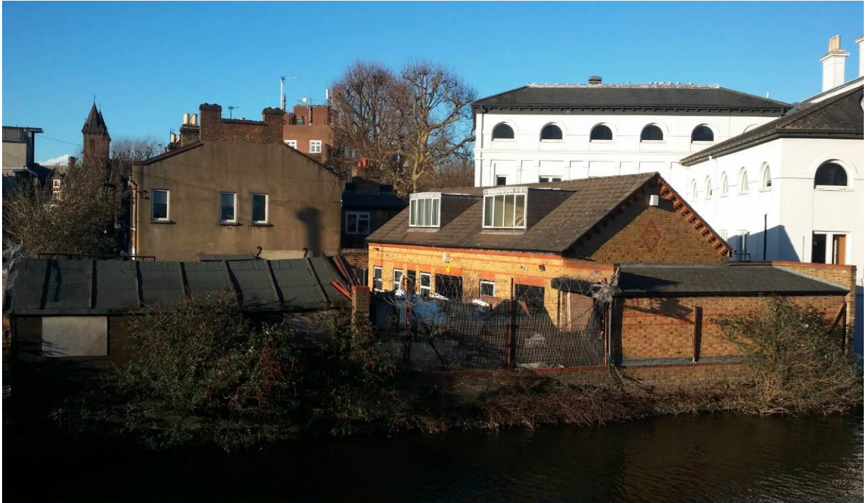
Application site as seen from opposite side of Grand Union Canal
